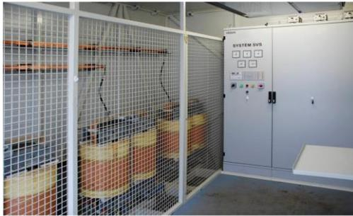
Fig.7. The VSS system of the three-phase earth fault current compensation, charging current elimination and phase voltage symmetrization in a 6 kV industrial network.
